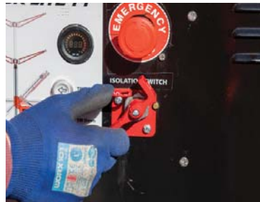
Isolation switch in OFF position
